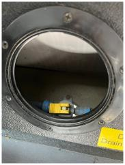
The yellow button is the cut off valve. When it is horizontal like this the pipes are locked and you can fill up the tank with water. Replace the cover.
