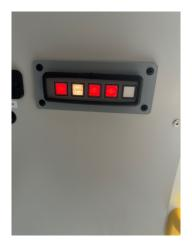
The PUMP button must be pressed for the water pump to work and get water to the taps and toilet flush. The LIGHTS is self-explanatory!
